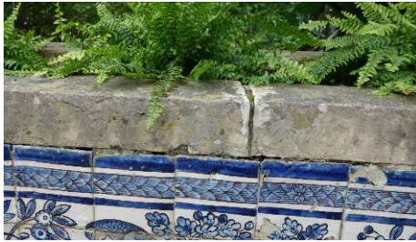
c. Open masonry joints.
