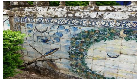
b. Panel fracture – masonry wall rotation.
