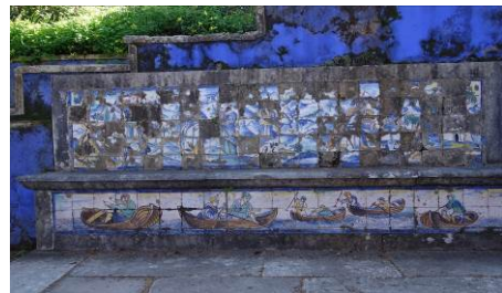
d. North side exposure deterioration.
