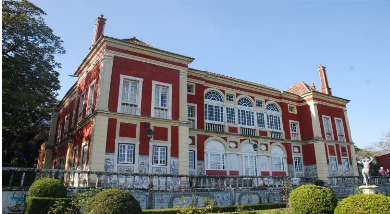
Figure 6 – East façade with enclosed loggia and gallery.
