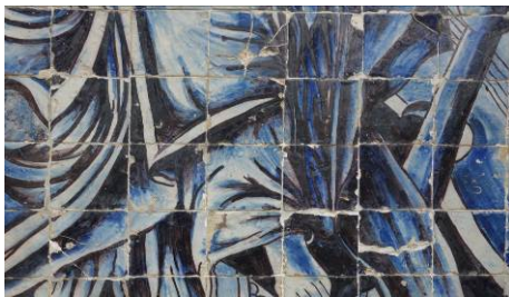
e. Surface cracking / glazing release.
