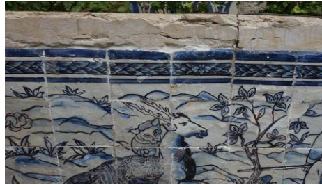
d. Joint closure (maintenance).
