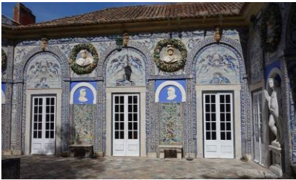
d. Dining Room doors.
