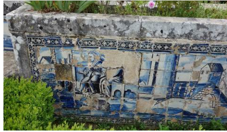
b. Humidity/ water infiltration.
