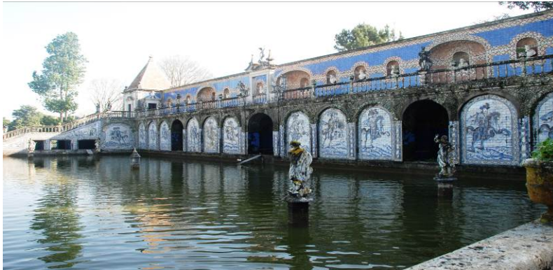
Figure 16 – The King's Gallery and the Large Water Tank.
